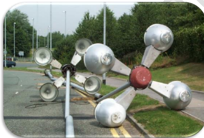
Figure 9.4 Maintenance of high mast lighting
