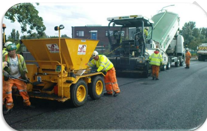
Figure 9.1 Carriageway resurfacing
